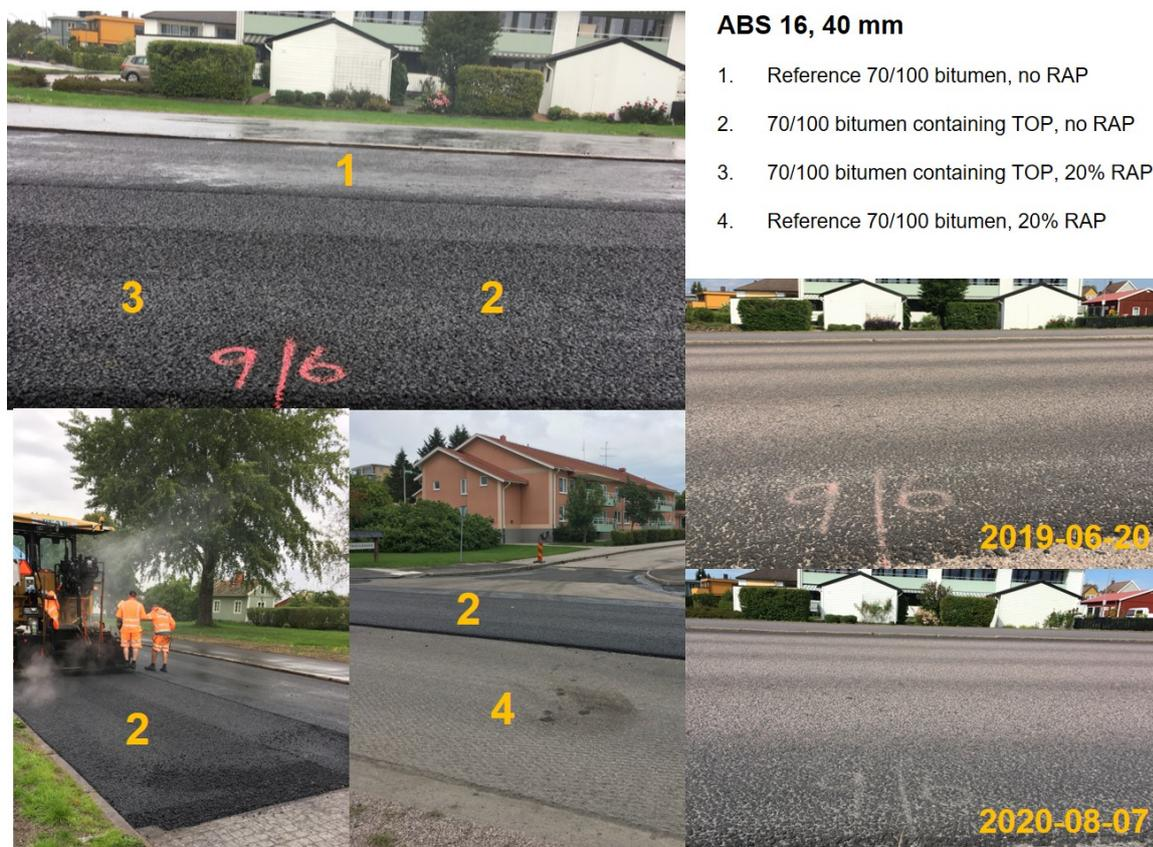
Figure 1. Field trial of bitumen containing TOP and performance follow up
