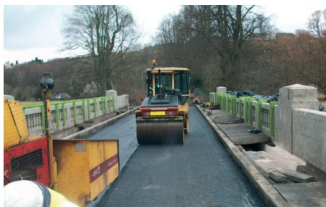
Use of the Cemex lower temperature asphalt meant that three layers could be placed within normal working hours during a single day.
