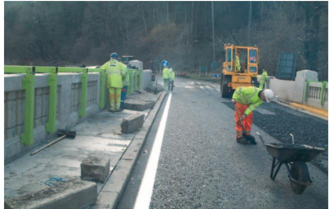
In the event, the base course asphalt supplied to Inchbonny gave no problems at all: it fulfilled all requirements in terms of workability and compaction, speed of laying and end performance. Everyone was pleased with the result.
