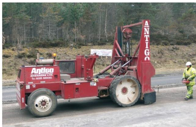
the concrete. The micro cracks subsequently act to take up thermal and traffic movement, allowing the concrete to become structurally part of a flexible composite pavement. The concrete is left, to become a useful contributor to the structure, instead of being wasted.
