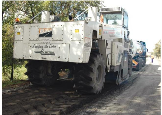
This extra aggregate was laid on top of the road surface and milled in during the pass of the Wirtgen 2500 Recycler. The amount of additional bitumen required was determined at 2.5 mass%, with 2% added water and 1% cement.
